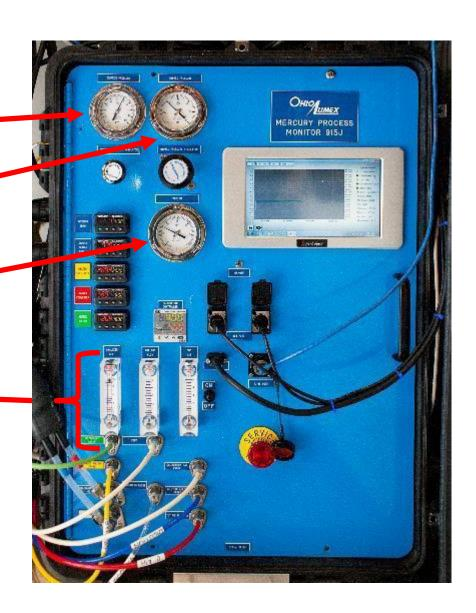
Before beginning work on the head, make sure to pull the Service Button on the bottom center of the console to cut air to the system!
